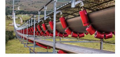
Standing on a ropeway 7,2 km long and up to 36 m high, this unique conveyor system transports 1,500 tph of limestone and clay from the quarry to Lafarge-Holcim's cement plant, while crossing valleys and a dense vegetation without ever touching the ground.
